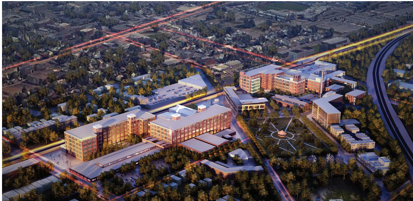
Electric Works, Fort Wayne, Indiana
